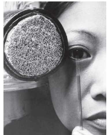
FIGURE 1.10 The small cable on the right contains 144 glass fibers and can carry more than three times as many telephone conversations as the traditional (and much larger) copper-wire cable on the left. (© Bettmann/CORBIS.)
